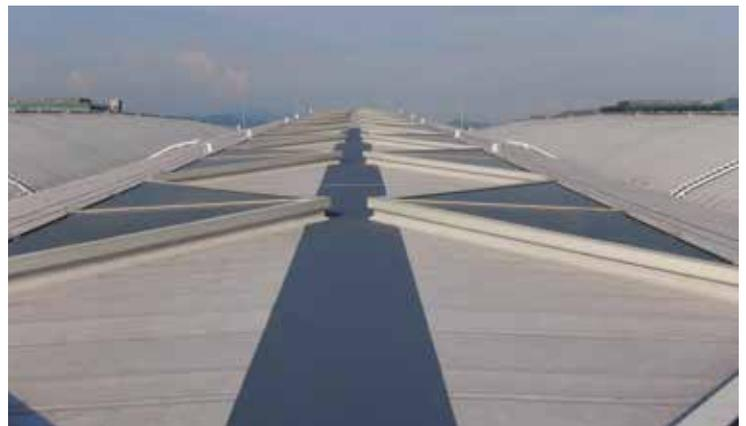
isting PVC sheet membrane waterproofing system of Terminal 1 roof. The loading of the additional waterproofing system to be imposed on the roof was not to exceed 2.5 kg/m<sup>2</sup>, while its fixing system needed to satisfy the design wind pressure with the highest figure 8.5kPa. Moreover, seam welding was mostly done by handheld welding guns instead of automatic machines. This was due to the dome shape profile of the roof where automatic machine could not be implemented.
