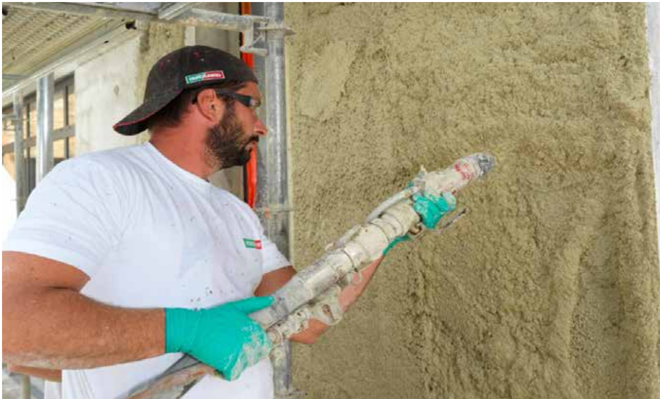
PARNATUR®, the first “easy-to-spray” thermal and phonic insulation hemp based mortar
