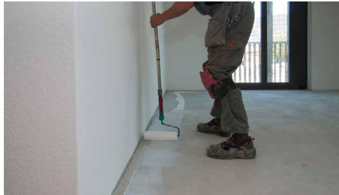
**Sika Primer MB and MR Fast** are 2 component epoxy based pre-treatments to enable successful wood floor bonding direct to the substrate (usually concrete or cement screed).
