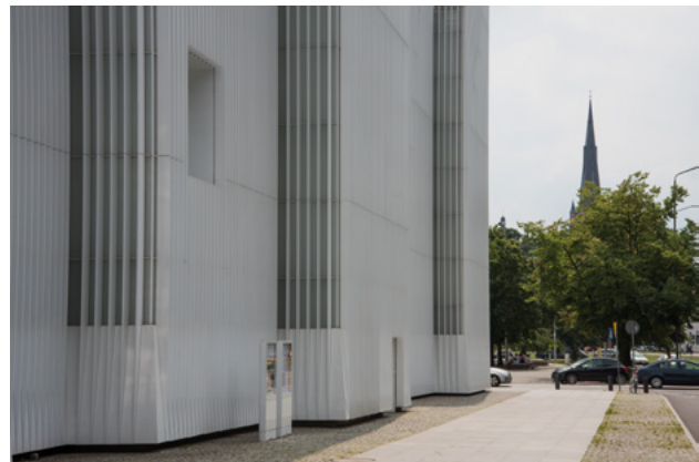
The graffiti protected facade of the Szczecin Philharmonic Hall.
