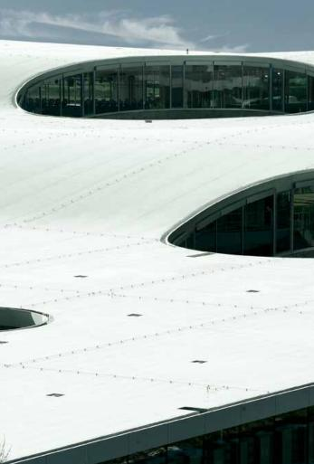
Curvatures and indentations, countersunk downspouts and lightning conductors applied directly to the roofing membranes. It was clear to me from the very start that in order to do justice to the architect's aesthetic will we would need an experienced partner.
