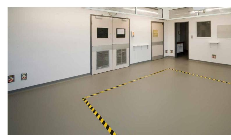
wet environment. This maintains the attractive, seamless finish and prevents the need for traditional and visually unappealing anti-slip treads that would also require a separate application. The system is equally suitable for new build and refurbishments.
