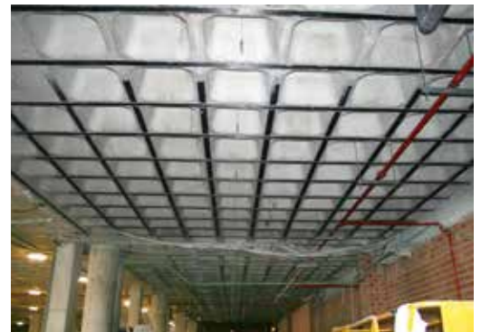
Structural strengthening
