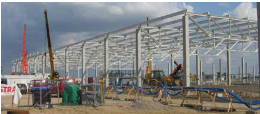
Steel structure protection and fire protection
