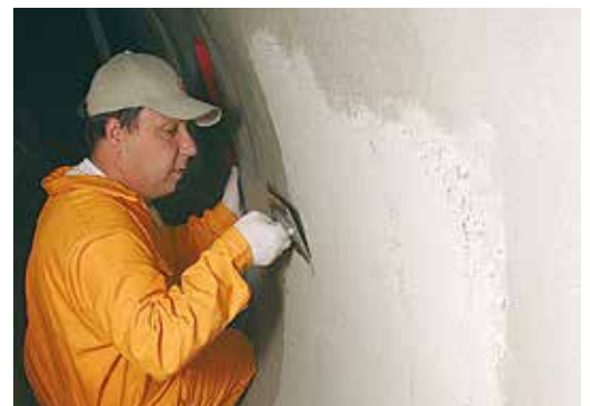
Concrete repair and protection
