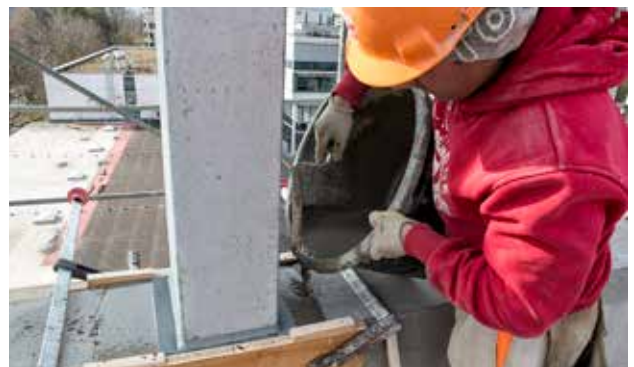
Grouting and fixing
