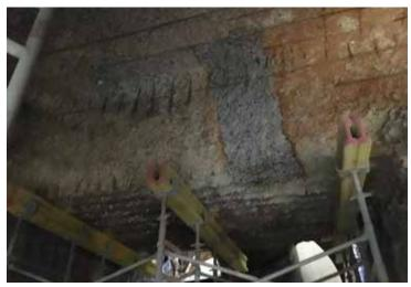
ing as a mould released agent was applied on the formwork. When the formwork was removed, immediate water jetting of the surface was done at ~150 bars to expose the aggregates, providing a perfect surface for the application of the biogenic corrosion protective mortar.
