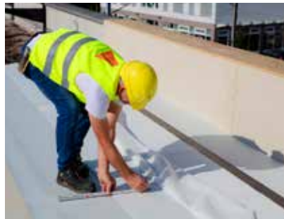
2. Mark position of upper parapet edge
