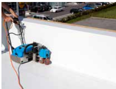
5. Final hot air seam welding
