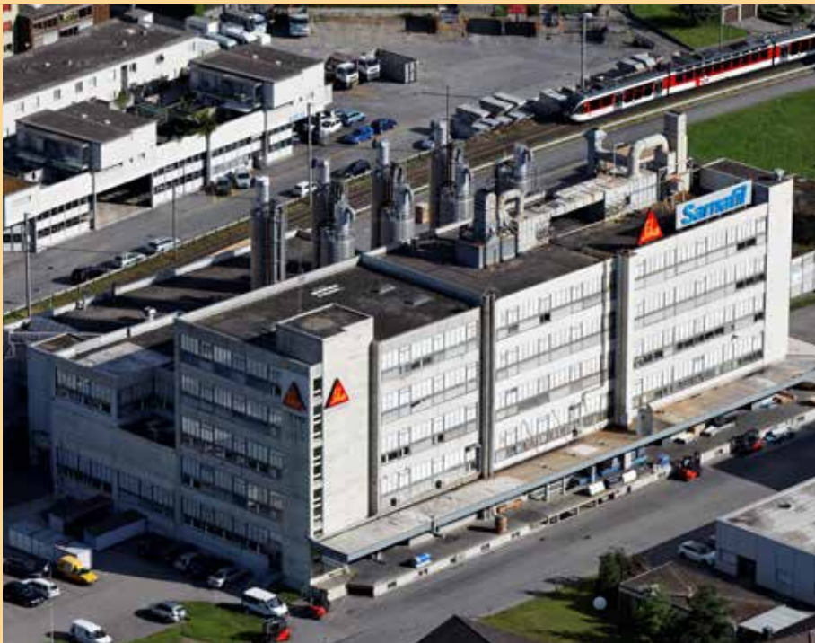
First Sarnafil® T roofing system installed in 1988 in Sarnen.
