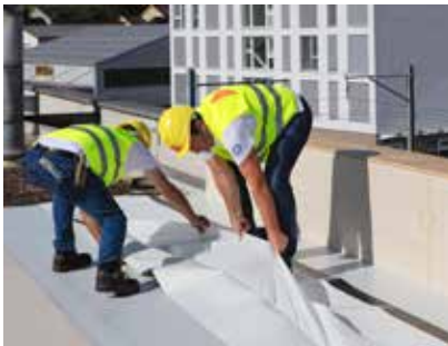
1. Remove Sarnafil® AT FSA P release liner
