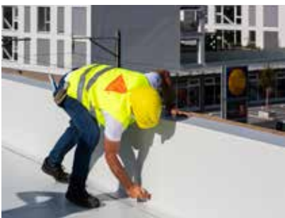
4. Press membrane in position with a suitable roller
