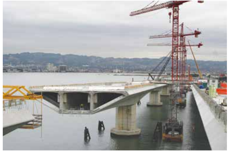
Construction of the skyway
