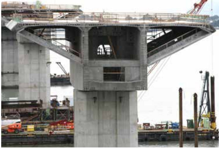
160 hollow steel-pipe piles
