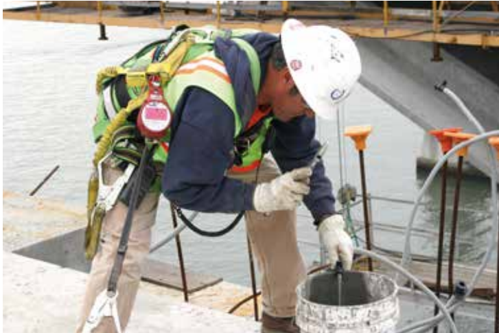
Grout coming out of the air pipe
