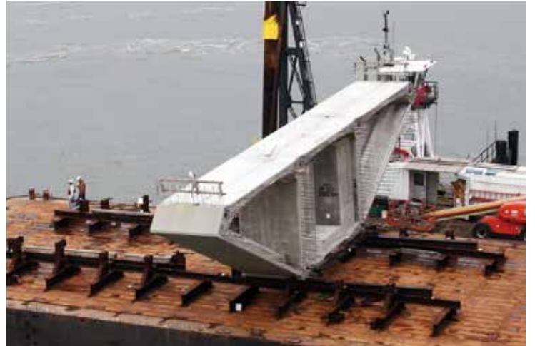
The precast element shipped to building site
