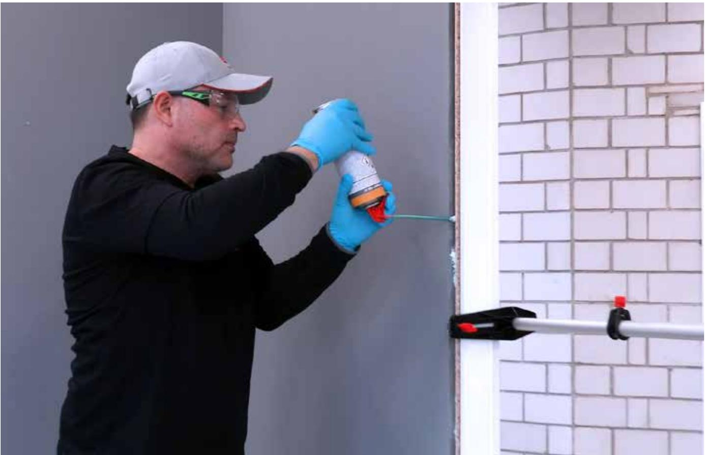
rigid foams are also ideal for the fast and secure installation and fixing of window and door frames, etc., where it easily expands and fills the gaps between the frames and the structure, as well as efficiently sealing and insulating all around the frames at the same time.
