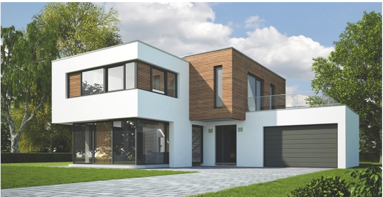
A fasthouse construction from Ireland where Sika products have been used in the modular construction.
