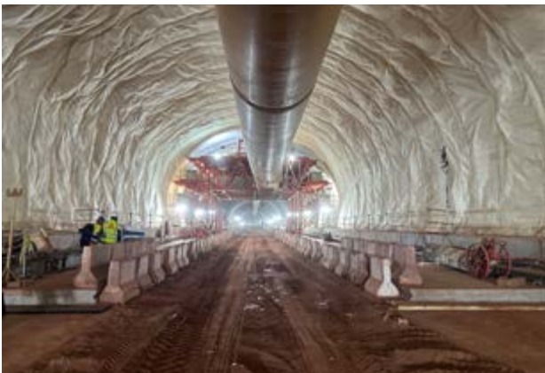
Mined Tunnel (drained), Saudi Arabia, SikaProof®-110, 1,000,000 m 2
