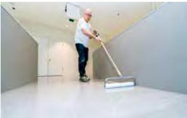
STEP 5. The finishing touch is the application of a transparent or pigmented topcoat. Typically this step involves a roller or spray application. The topcoat secures the desired final design, and adds friction and wear resistance qualities to the buildup.
