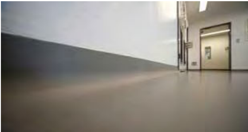
Coving Solution with Sikafloor® and SikaGard® WallCoat.
