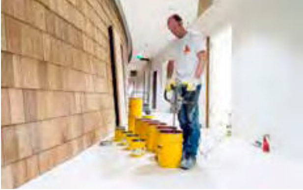
STEP 1. After inspection and preparation of the subfloor by cleaning (and if needed shotblasting, grinding, sanding and/or leveling), we will start mixing our liquid materials.
