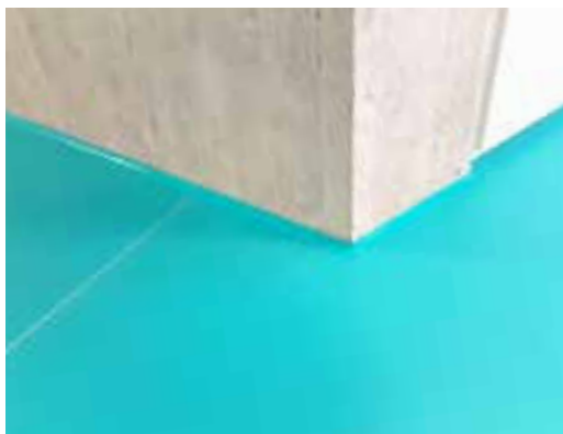
Sikafloor® Joint Solution with Sikaflex® PRO-3.
