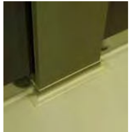
Floor-Wall Connection with Sikafloor® and SikaGard® WallCoat.
