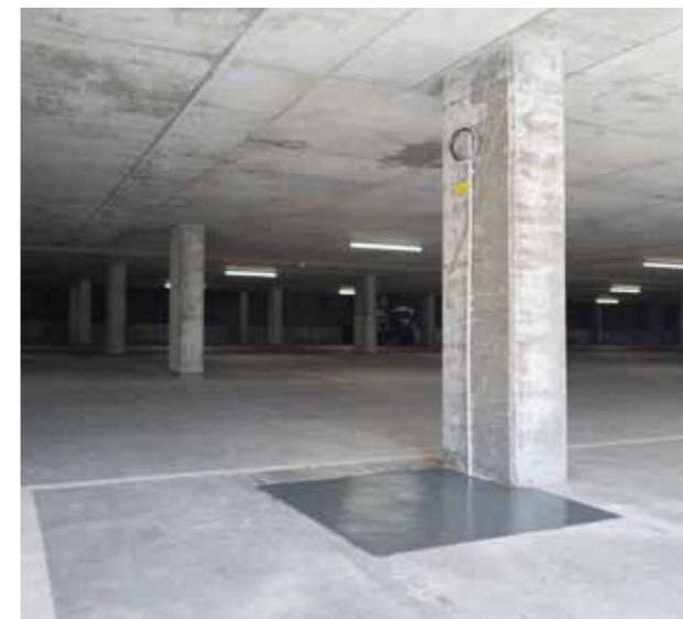
Typically, Sikafloor® system does not allow vapour diffusion, so the concrete CAN NOT dry out.
