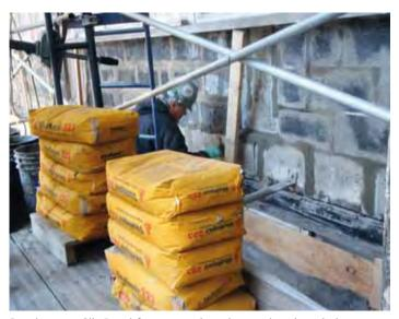
Repair mortar SikaRepair®-223 was selected to repair and patch the mortar joints, cracks and voids of the existing concrete wall structure to provide a uniform substrate before applying the membrane.
