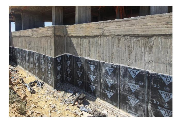
**SikaShield® W IS AN INNOVATIVE SOLUTION** that combines the use of a polymer-modified bituminous membrane with a specially modified cement-based adhesive, ensuring fully bonded and reliable waterproofing of the substrate.
