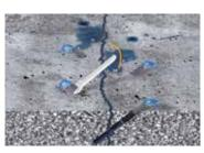
**2.** Install the mechanical packers. Tighten the mechanical packers so that they can withstand the maximum injection pressure.
