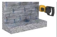
Drill holes for the mechanical packers through the leaking building component at a spacing of 30 - 50 cm as shown in the picture.
