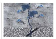
**3.** Fix the non-return valve on the first packer and start the injection process.
