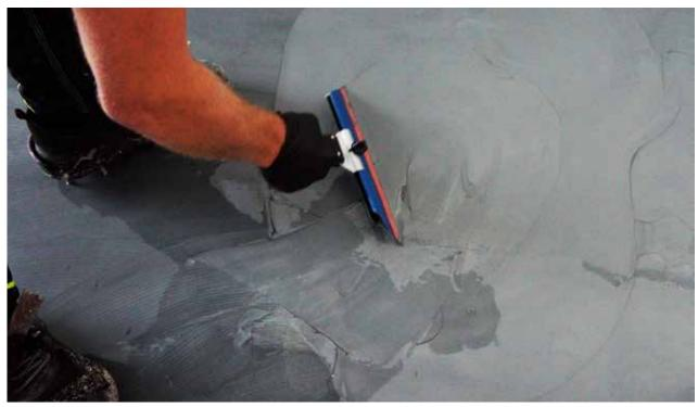
Sikafloor®-3000 FX is distributed on the surface and then reworked with different tools. Depending on the tool used, the floor gets its individual look.
