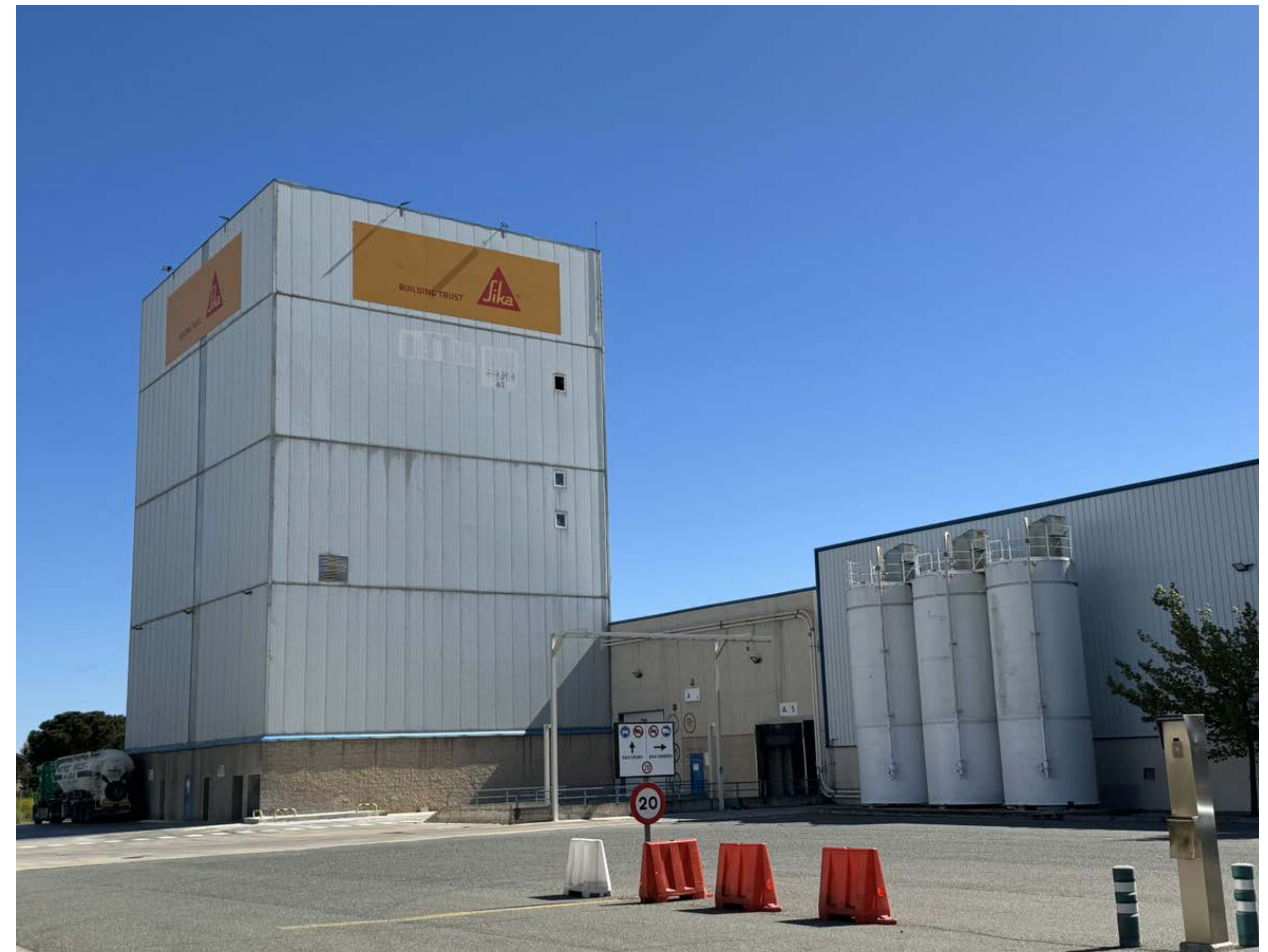
The former MBCC plant in Cabanillas del Campo: the joint expertise and knowledge of the Sika and MBCC teams led to a new level of operational excellence.
