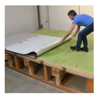
Fold half of the membrane back. Cut release-liner over the width of the membrane.
