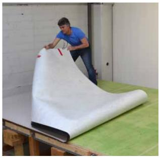
Remove release liner on half of the membrane by drawing off. Adhere the membrane to the substrate. We recommend using a brush or a putty knife to prevent blisters. Execute the same procedure on the other half of the membrane.
