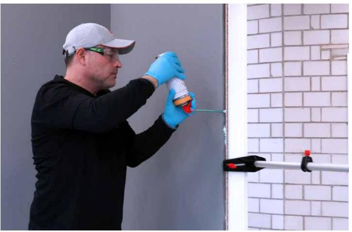
rigid foams are also ideal for the fast and secure installation and fixing of window and door frames, etc., where it easily expands and fills the gaps between the frames and the structure, as well as efficiently sealing and insulating all around the frames at the same time.
