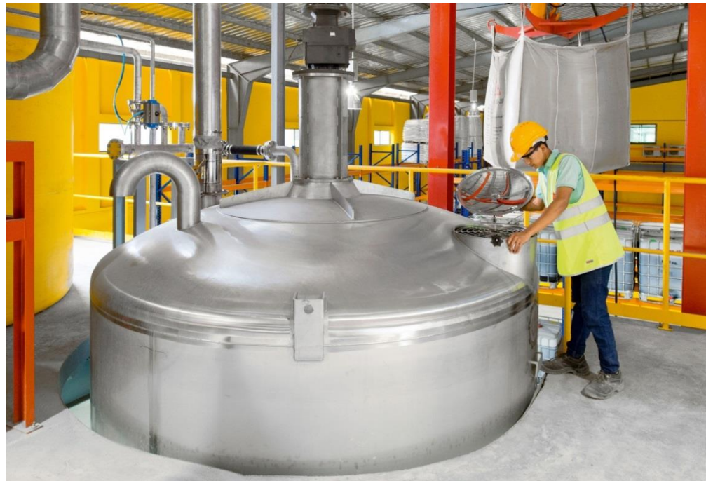
Sika Myanmar production facilities
