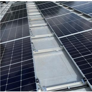
Due to the M12 inside thread, it is easy to assemble a broad range of solar construction onto the SikaRoof® Anchor System.
