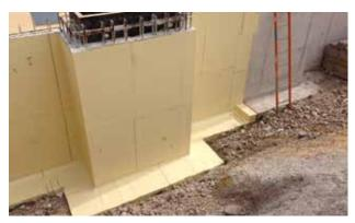
Open excavation with protrusion slab to wall: The complete structure is sealed with SikaProof® P.
