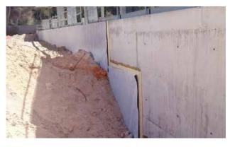
For open excavations: The protection of the SikaProof® membrane is mandatory, especially regarding the backfilling.
