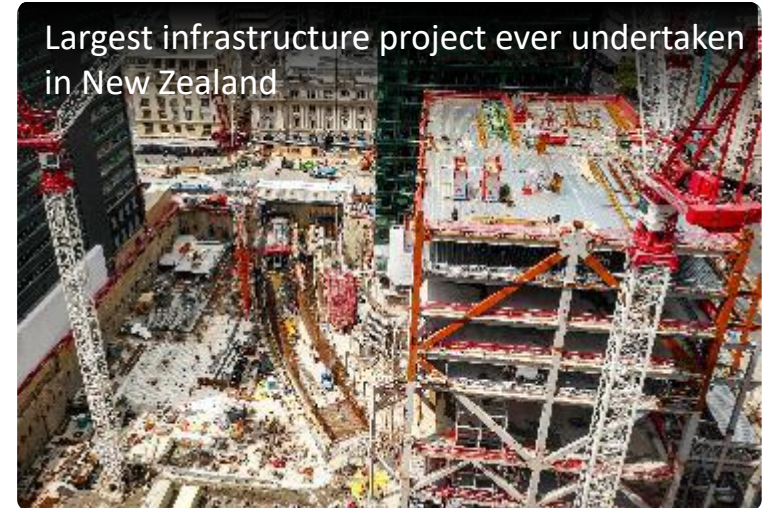
City Rail Link, Auckland, New Zealand
