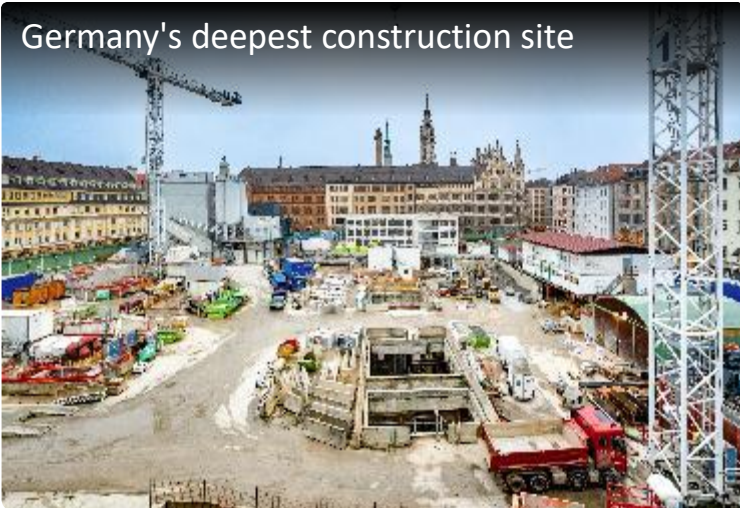
Marienhof S-Bahn Station and Line, Munich, Germany
