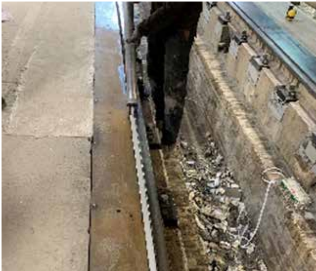
Casting of sealant Sikaflex®-406 KC along the rail
