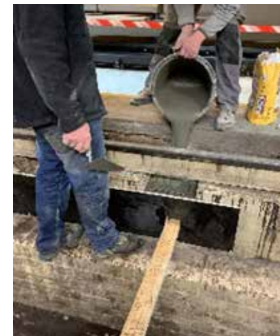
Creation of supports for steel baseplates
