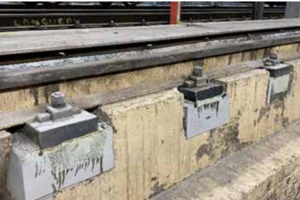
Grouted steel plates
