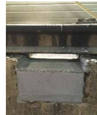
New cast supports using Sikagrout®-238 Chargé
