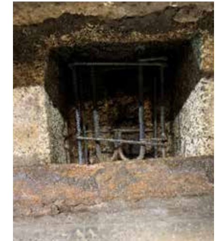
Reinforcing bars for connection to the existing concrete substrate
