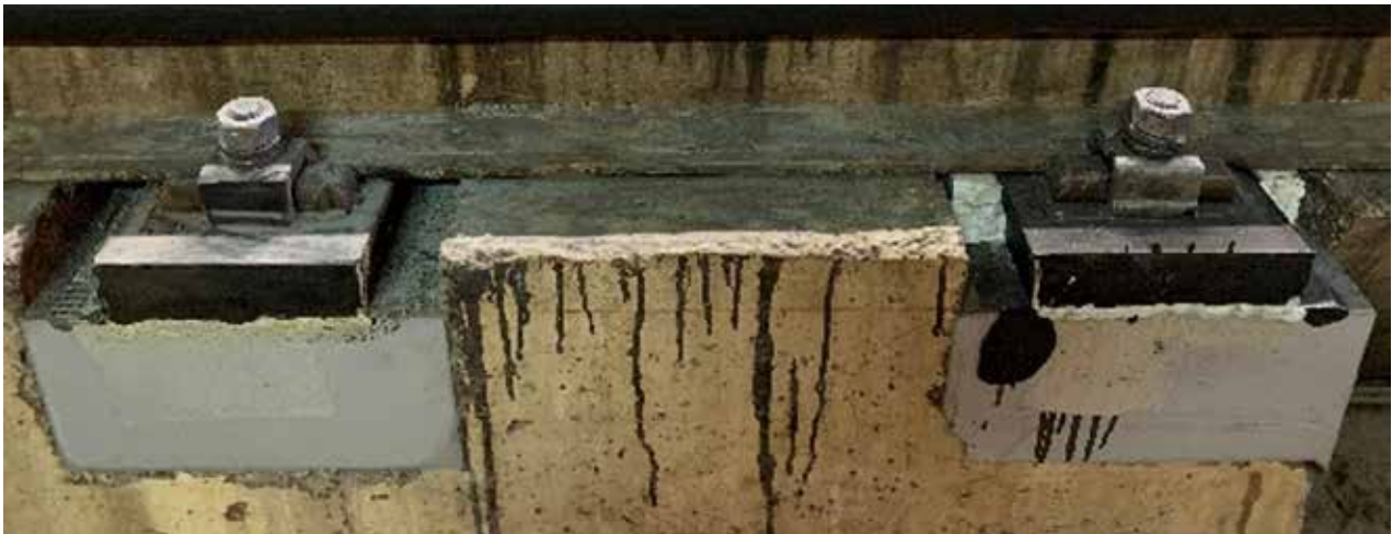
Completion of the work
