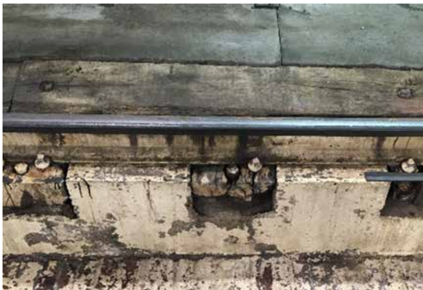
Existing old wooden sleepers and anchorages
