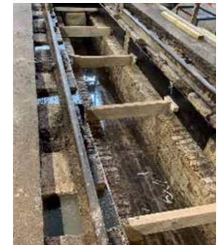
Reinforcing bars for connection to the existing concrete substrate
