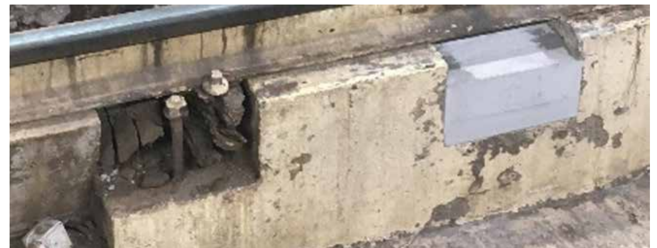
The old wooden sleeper and the new sleeper made of Sikagrout®-238 Chargé
