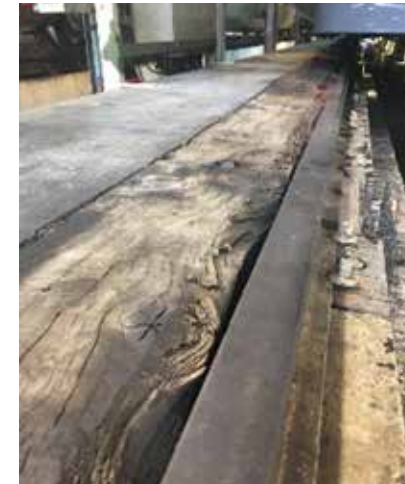
Side of the track made of wooden pieces
