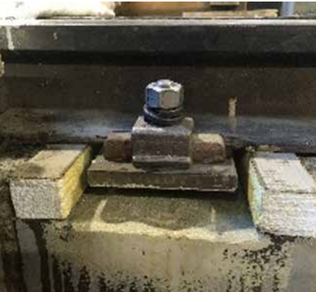
Formwork around steel baseplate
