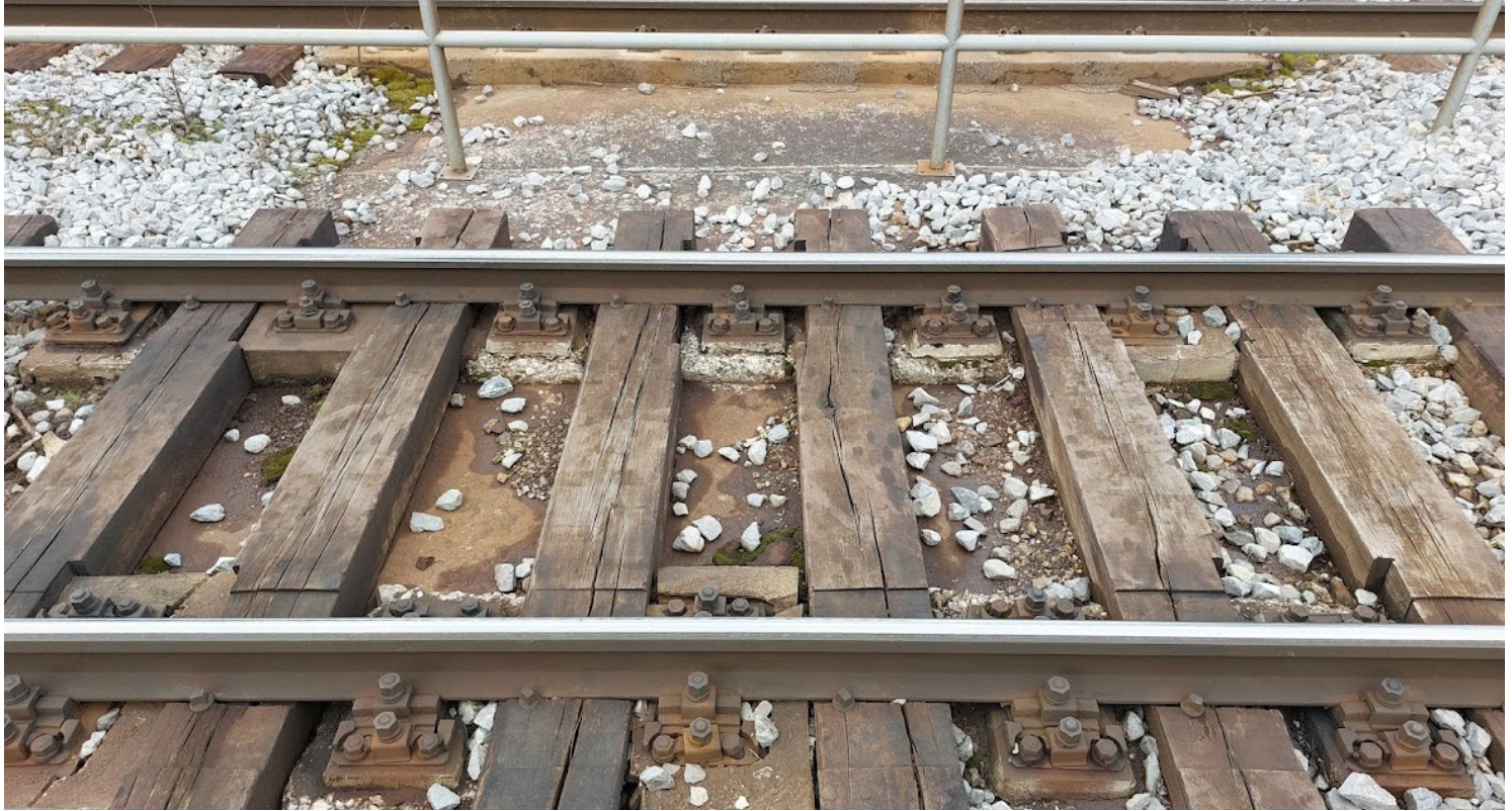
The initial condition of the foundations
