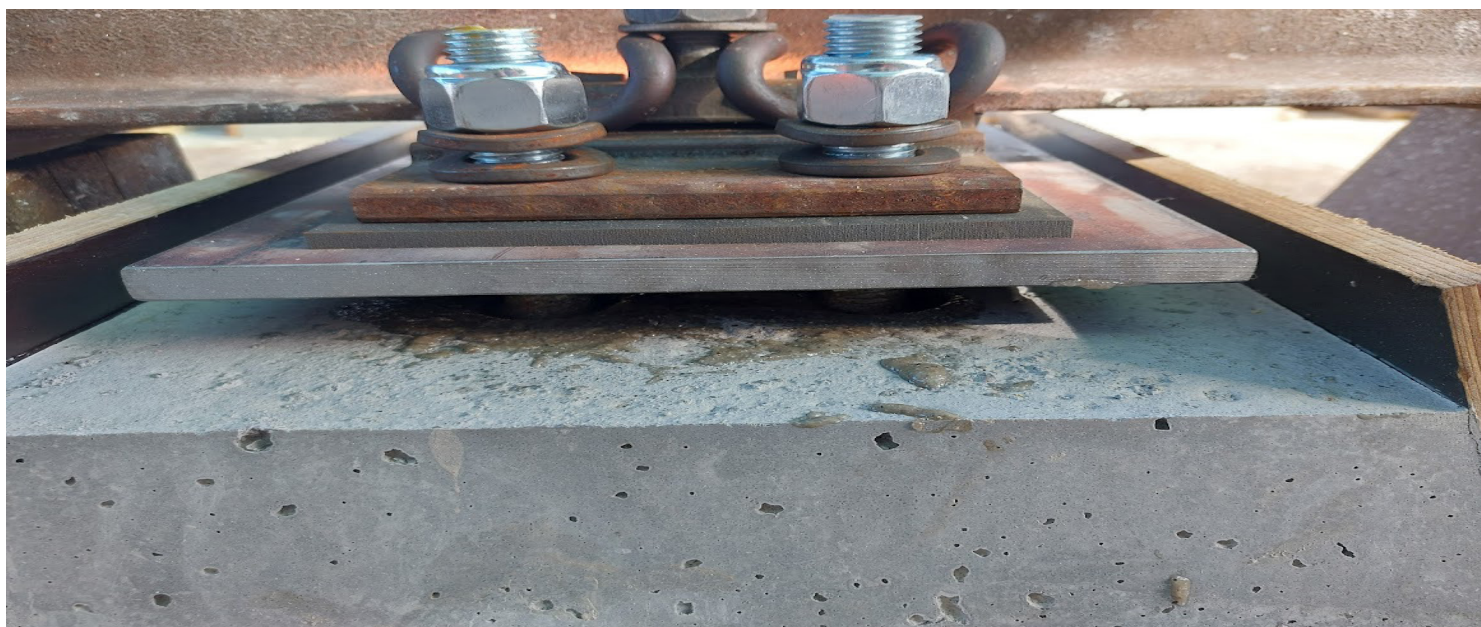
Space for Icosit installation.
