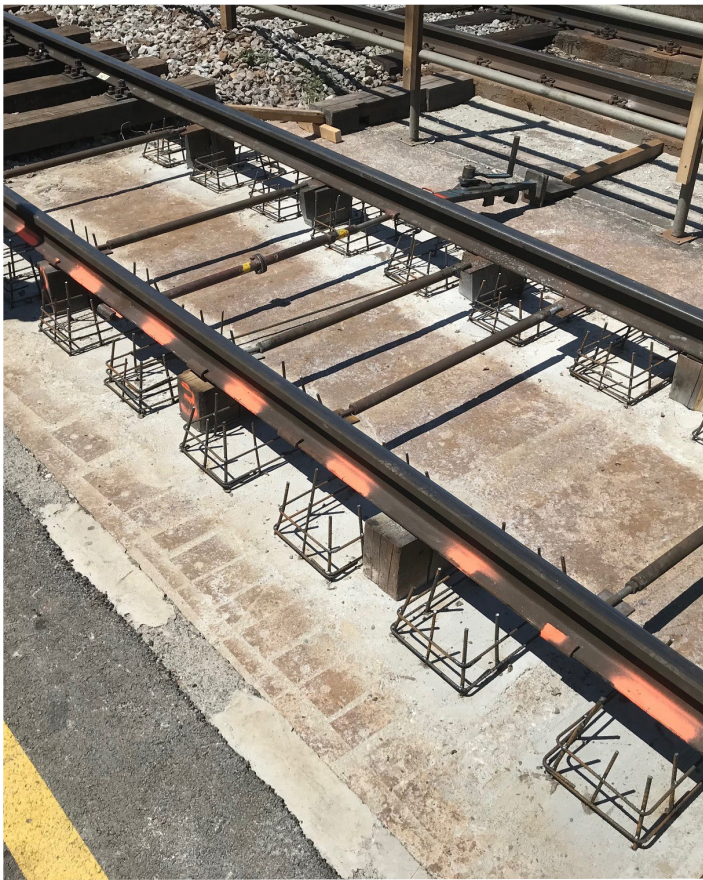
Preparation of the surface by complete removal of the old foundation, sandblasting and leveling with Sikadur®-12 Pronto.
