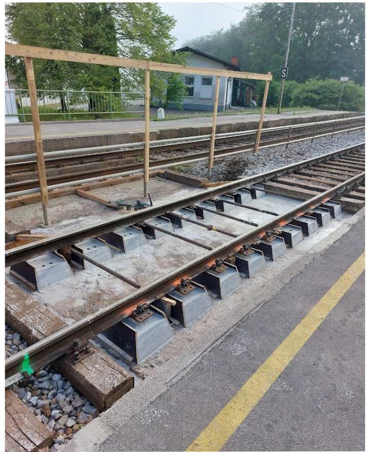
Production of formwork and installation of Sikadur®-12 Pronto in 2 phases. Drilling for anchoring the threaded rods.
