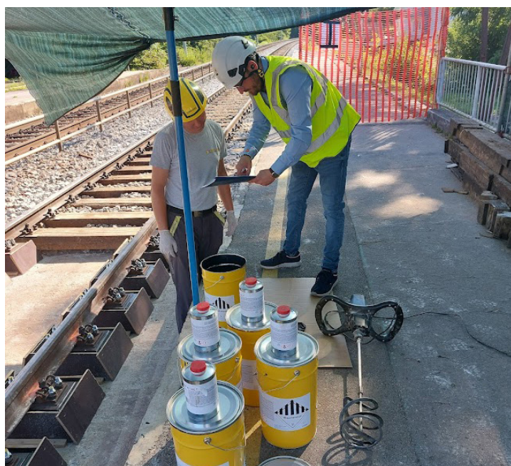
Advice before starting mixing and application.
