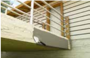
Increase the concrete cover of existing concrete structures -> Restoring Pasivity
