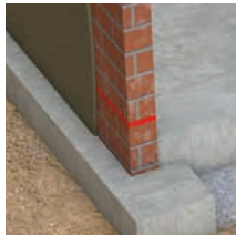
3. DAMP PROOF COURSE (DPC) / EXTERNAL INJECTION to prevent moisture from rising through masonry as a result of capillary action
