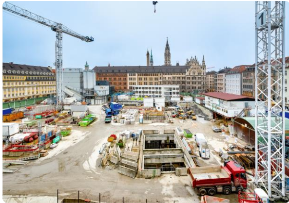
Marienhof S-Bahn Station and Line, Munich, Germany
