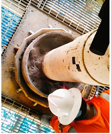
The installation included primary and secondary grout inlets, with all operations performed by a team of twelve certified offshore grouting personnel working 12-hour shifts. Quality control was ensured through continuous monitoring of grout volumes, temperatures, and flow rates, as well as the casting and third-party testing of grout cubes for 28-day compressive strength verification.
