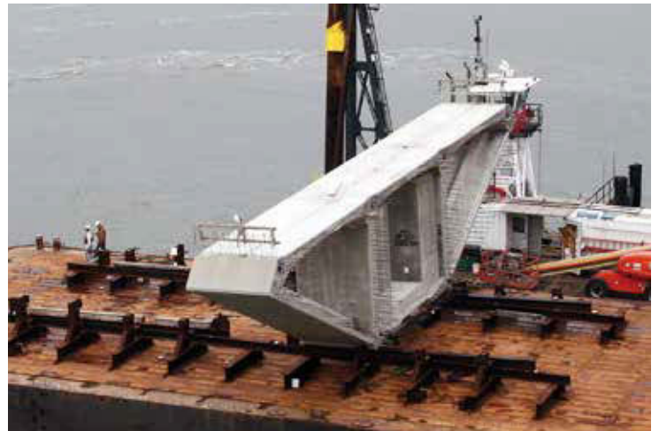
The precast element shipped to building site
