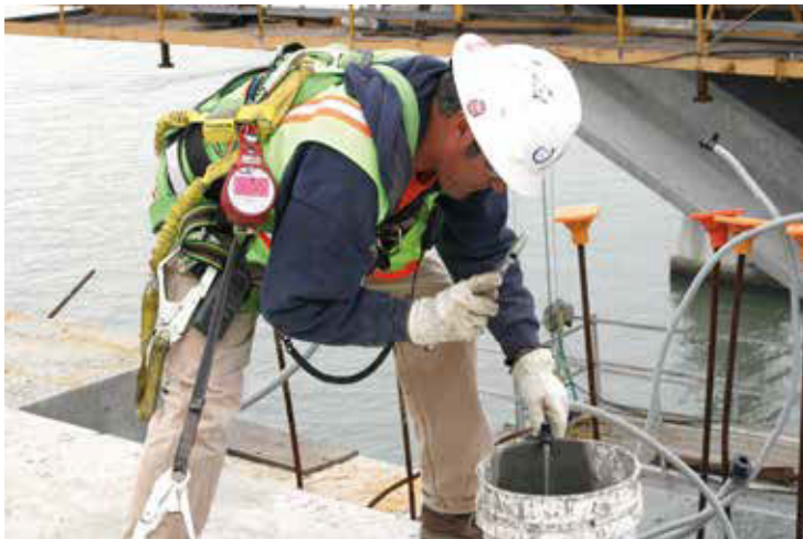
Grout coming out of the air pipe
