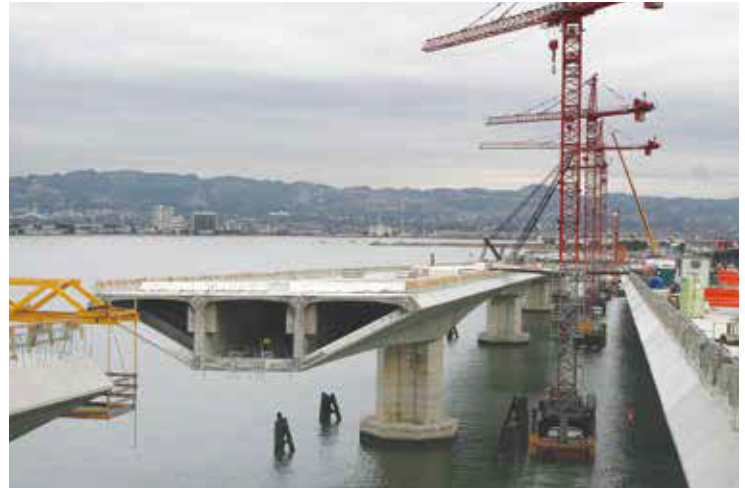
Construction of the skyway
