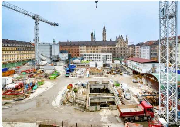
Marienhof S-Bahn Station and Line, Munich, Germany
