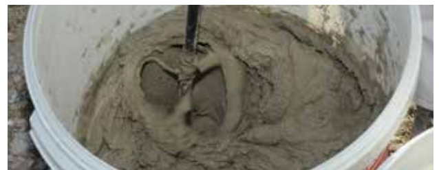
Mix MonoTop®-3200 Grid mortar.
