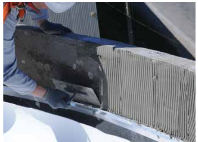
Apply first layer of MonoTop®-3200 Grid mortar.
