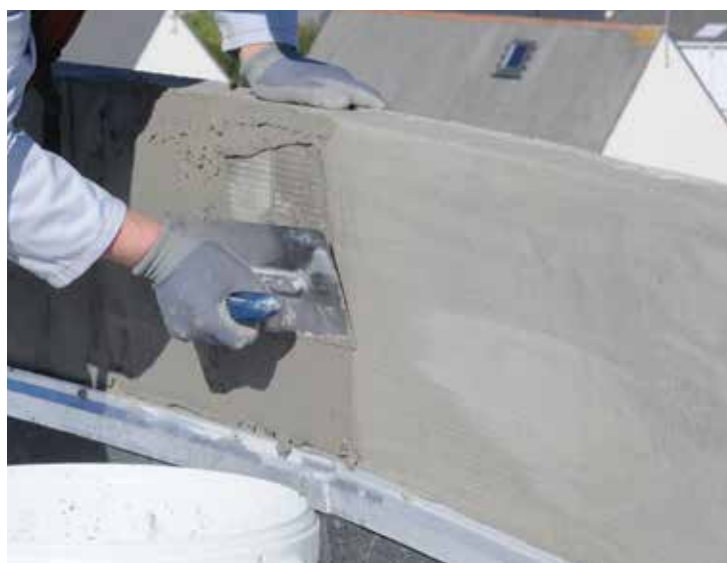
Apply second layer of MonoTop®-3200 Grid mortar.
