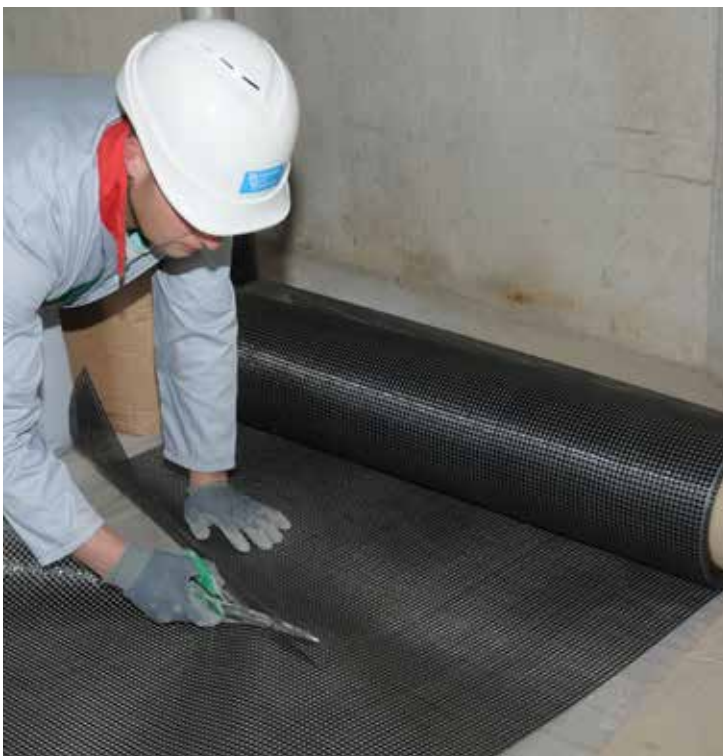
Cut Sika CarboDur® 300 Grid.
