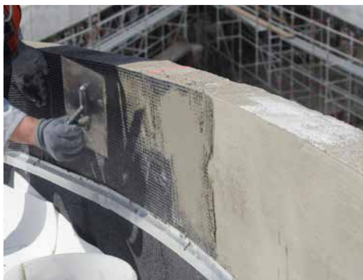
Sika CarboDur® 300 Grid is then embedded in the mortar.
