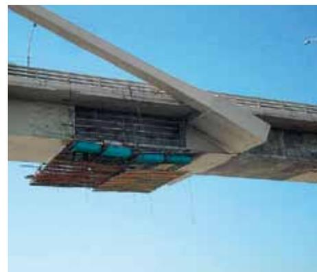
process. Sika's products and systems such as corrosion inhibitors, repair mortars, protective coatings and carbon-fiber-based strengthening systems, nonetheless allowed the full eco-efficient rehabilitation of the bridge such that only routine maintenance will be required in the decades ahead. ■
