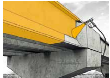
Machine applied using airless spray.
