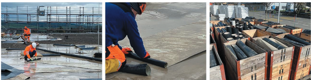
Figure 2. Different phases of the material reclaiming process: pre-cleaning, cutting, rolling, and storing.
