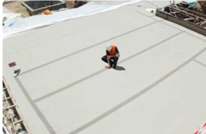
Below Grade Waterproofing
