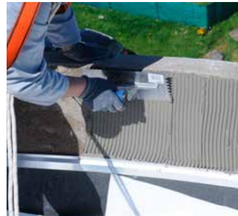
The mortar is applied with a notched trowel.
