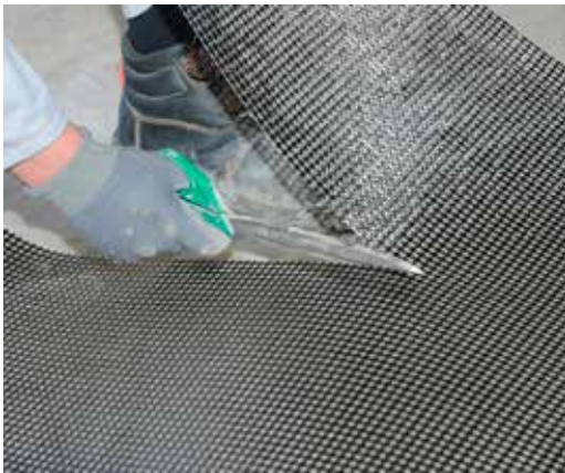
Cutting of reinforcements before installation.
