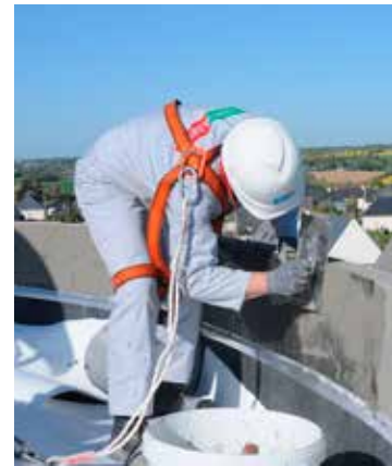
The CarboGrid is placed.
