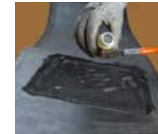
Clean and degrease the surface using SikaBond® R&B-100 Cleaner
