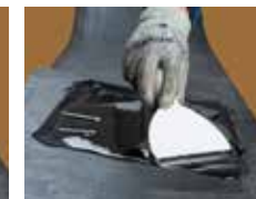
If necessary, spread the still liquid product evenly over the area to be repaired (using the spatula provided)
