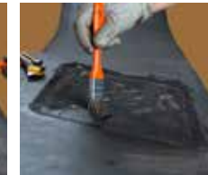
Apply SikaBond® R&B-100 Primer on to the cleaned surface in a thin film
