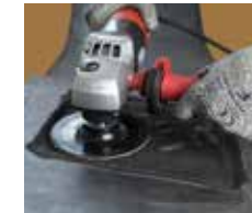
Grind away any damaged rubber, without tearing the textile carcass, leaving as much sound rubber as possible
