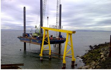
The steel jacket structure was anchored to the seabed using a technique known as rock socket grouting. Piles were inserted into 30 meters deep pre-drilled rock sockets. Specialist contractor FoundOcean Ltd. utilized its Super Pan Mixer, which doubles grout output rates compared to conventional high-strength grout mixers. 909 metric tons of SikaGrout®-9500 was pumped through a flexible hose and injected into the annulus, with grouting continuing until high-quality returns were observed.
